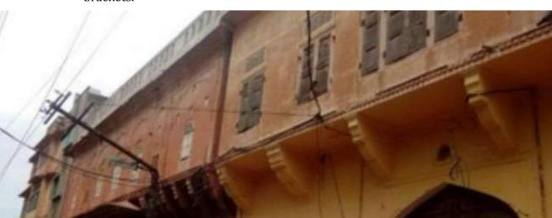
❖ Jharokhas: These are partly projected balconies covered with oblong domes and pardiwalls on three sides and are generally fitted with small windows or Jalis, for light and ventilation.
