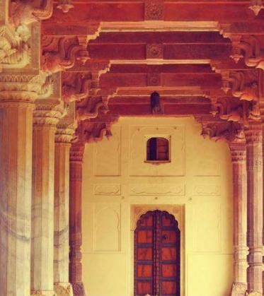
**Entrances:** Large opening like main entrance gates are spanned by cusped or pointed arches. Smaller openings are spanned by stone lintels.
